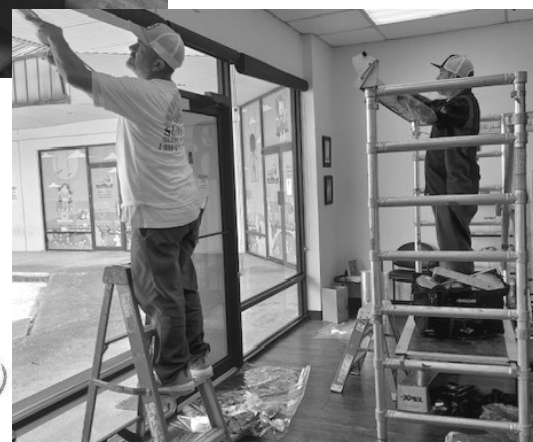
Security film being installed at the office
